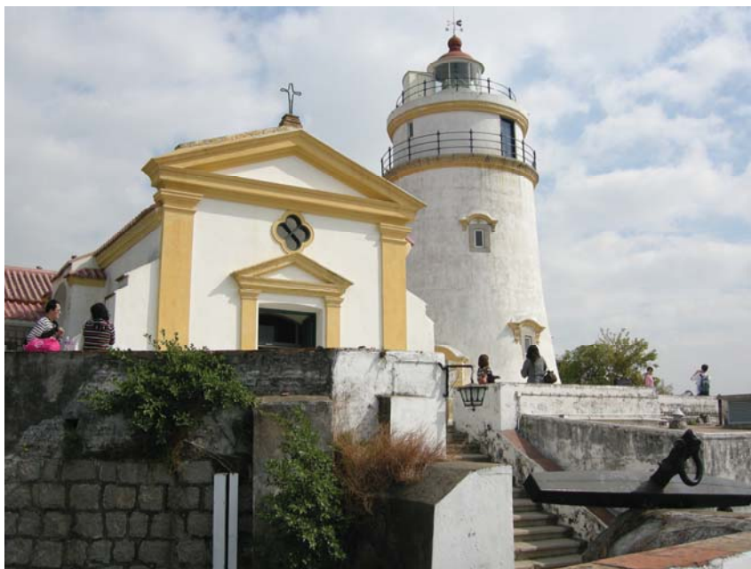
Figure 1: View Showing Guia Lighthouse within the Guia Fortress, at the Summit of Guia Hill
