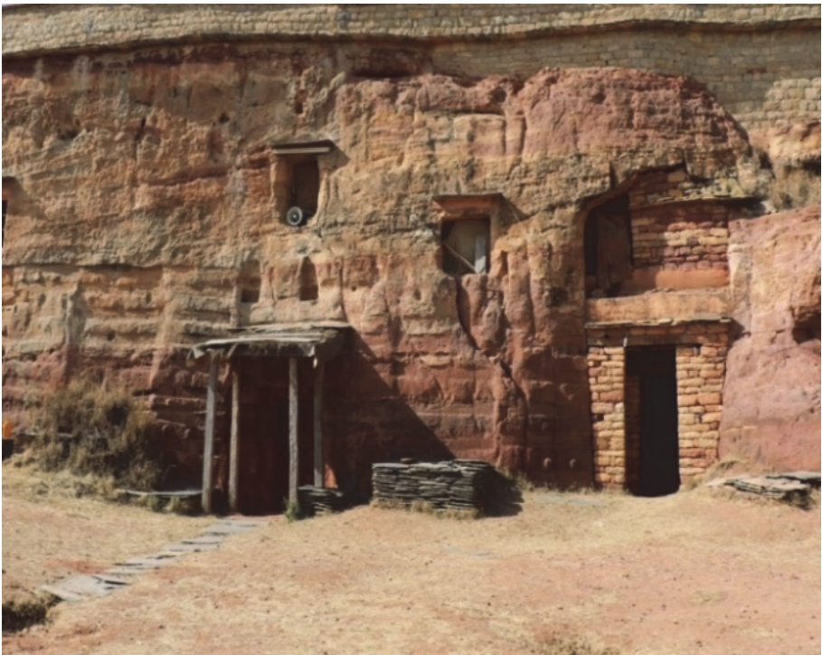
Fig. 2 The rock-hewn church of Däbrä Şəyon ( Abunä Abrəham ) from outside, photograph by Hagos Abrha, March 2018.
