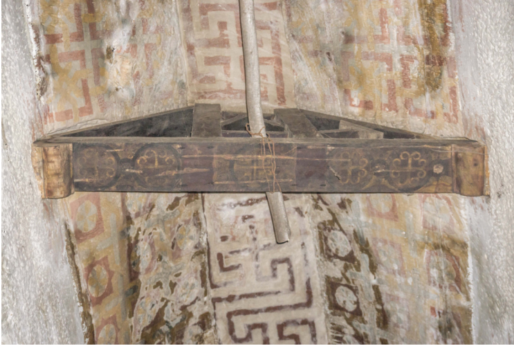
Fig. 14 G w ahgot Iyäsus, roof truss (photograph by the author, 2018).
